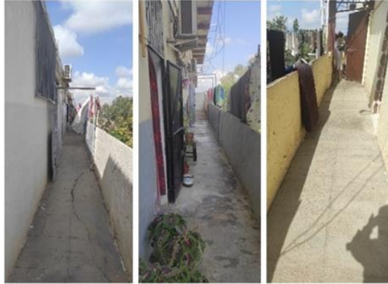
Fig. 6. Doors installed by residents on the corridors (Authors, 2023)
