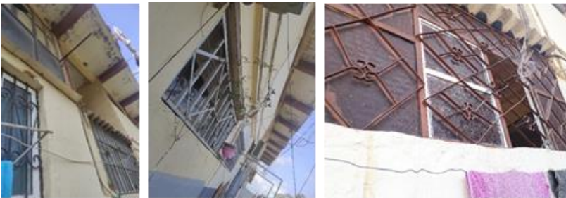
Fig. 10. The bars installed on the windows overlooking the corridor (Authors, 2023)
