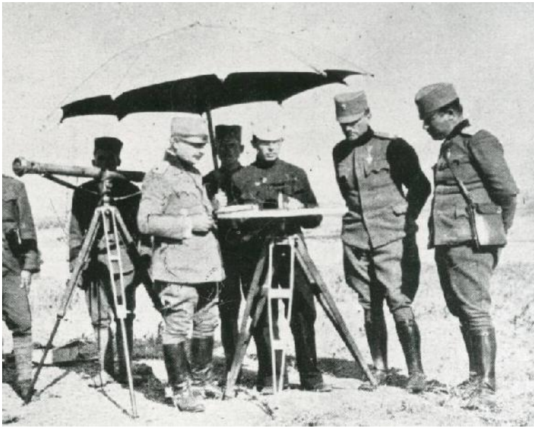
Fig. 4. Survey control, 1:50,000, cca 1923; Rostislav E. Tjabin at geodetic table, in the middle
