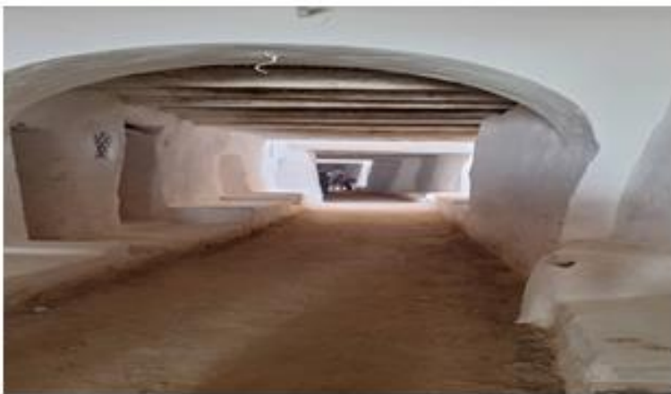
Fig. 6. Building materials with high thermal resistance (Jarad, 2024)
